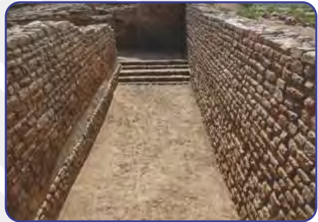
Covered drains along the roads, Mohenjodaro
